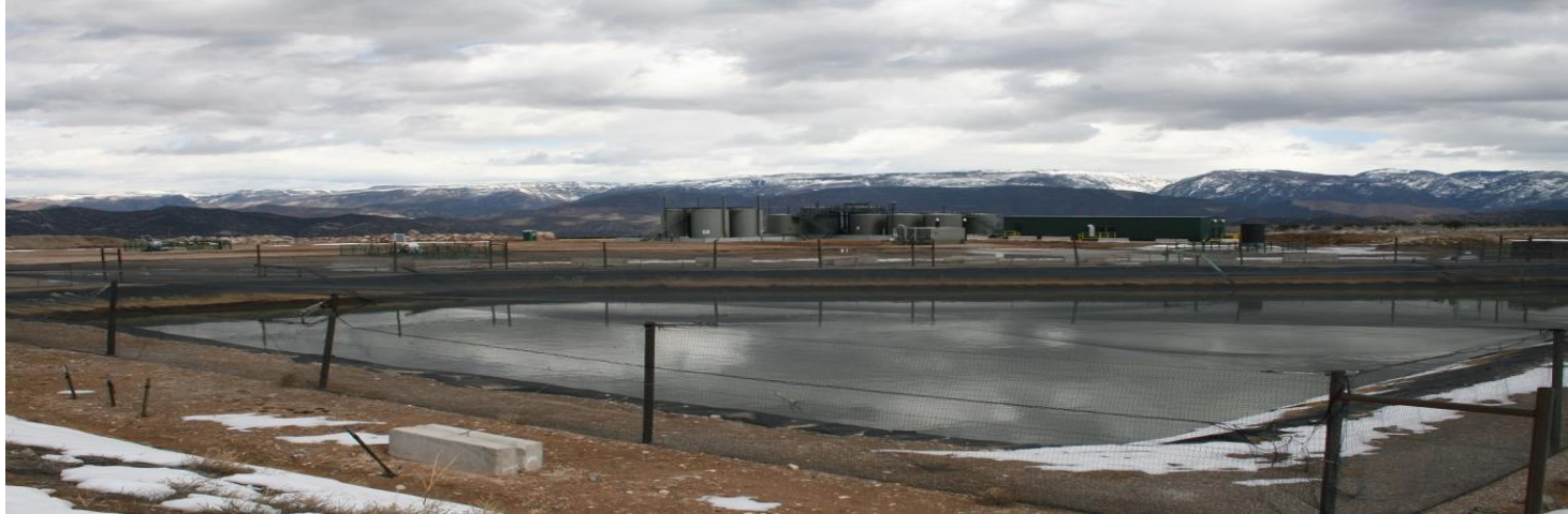
Pad 21A at Kokopelli Project
